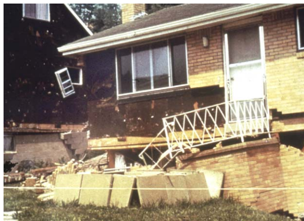
FIGURE 5 A house damaged by subsidence caused by the collapse of pillars in an abandoned underground mine.
