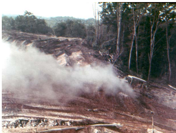
FIGURE 6 Excavation and extinguishment of a burning coal refuse pile.
