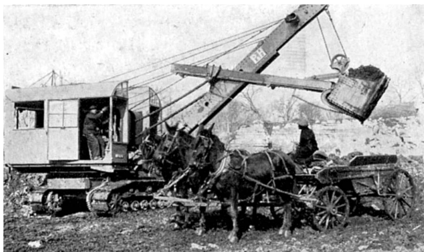
FIGURE 3 Early mechanized surface coal mining. A 1920s vintage P&H shovel loading in a coal wagon pulled by three horses. Photograph courtesy of P&H Mining Equipment, A Joy Global Inc. Company, Milwaukee, WI. Used with permission.
