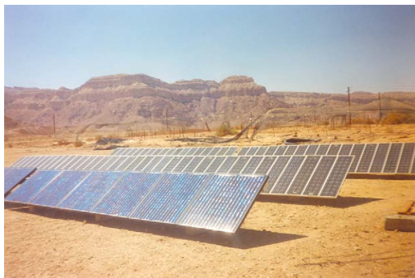
FIGURE 1 An array of photovoltaic panels at kibbutz Samar in the Negev Desert. Note the spacing between panels, necessary to prevent mutual shading and to allow access for cleaning. Photo courtesy of Bryan Medwed.
