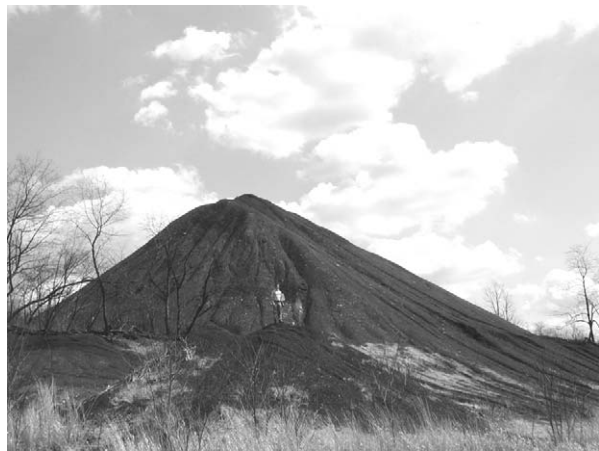
FIGURE 4 An abandoned coal refuse pile that leaches acidic drainage; many of these waste piles can be converted into a resource by burning the material in a fluidized bed combustion unit.
