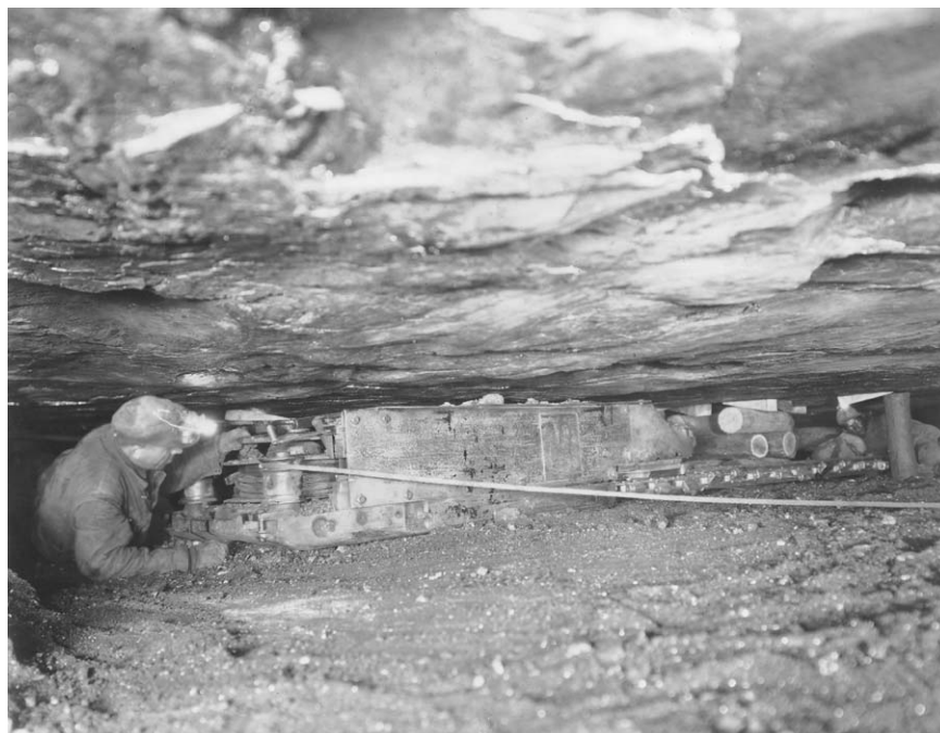
FIGURE 5 A major, highly successful advance in mechanizing underground coal mining: replacing manual undercutting by mechanical cutting. Jeffrey 24-B Longwall Cutter. Photograph and reproduction courtesy of Ohio Historical Society, Columbus, OH. Used with permission.
